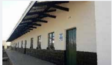
Sabiwa Primary Completed Block B
